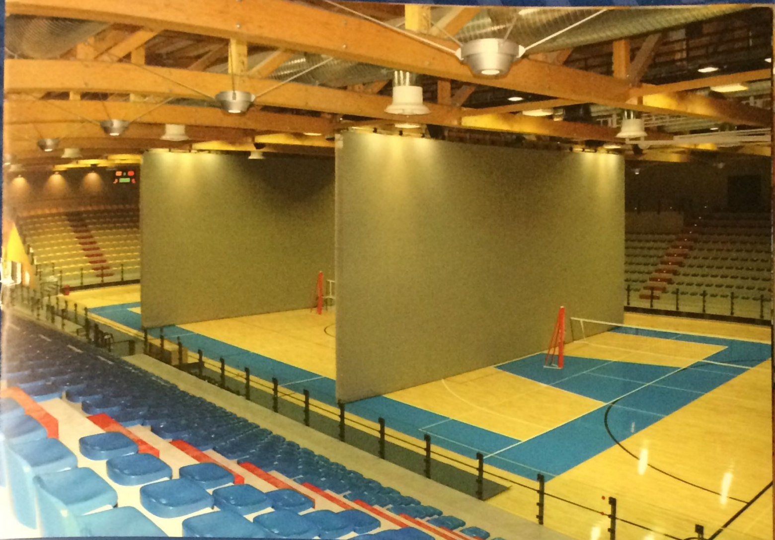
Paretazione del campo in tre settori / Automated partition walls to divide ground into three section
